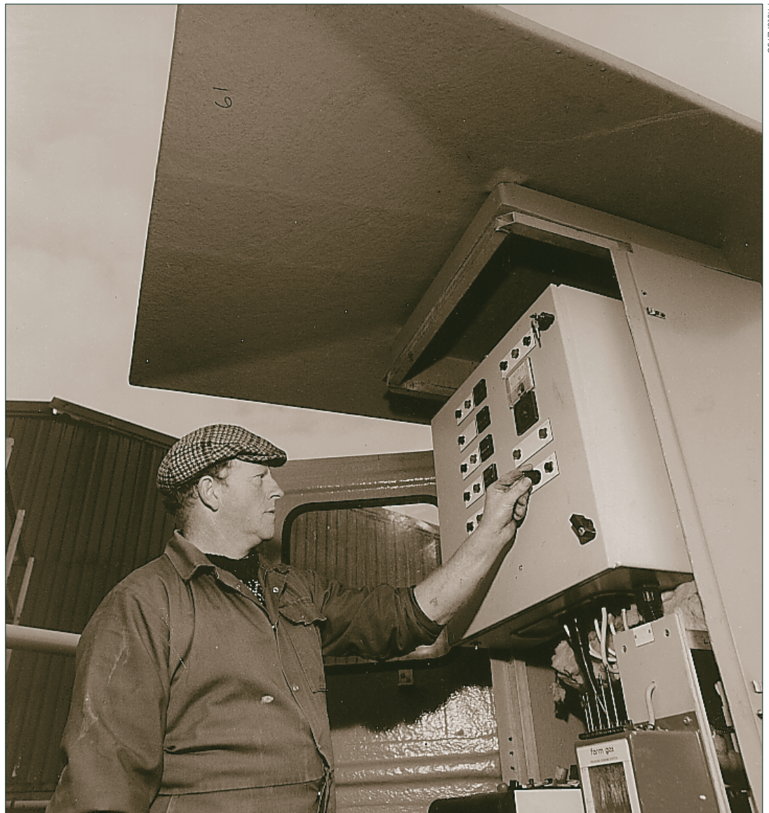
Digester control panel
