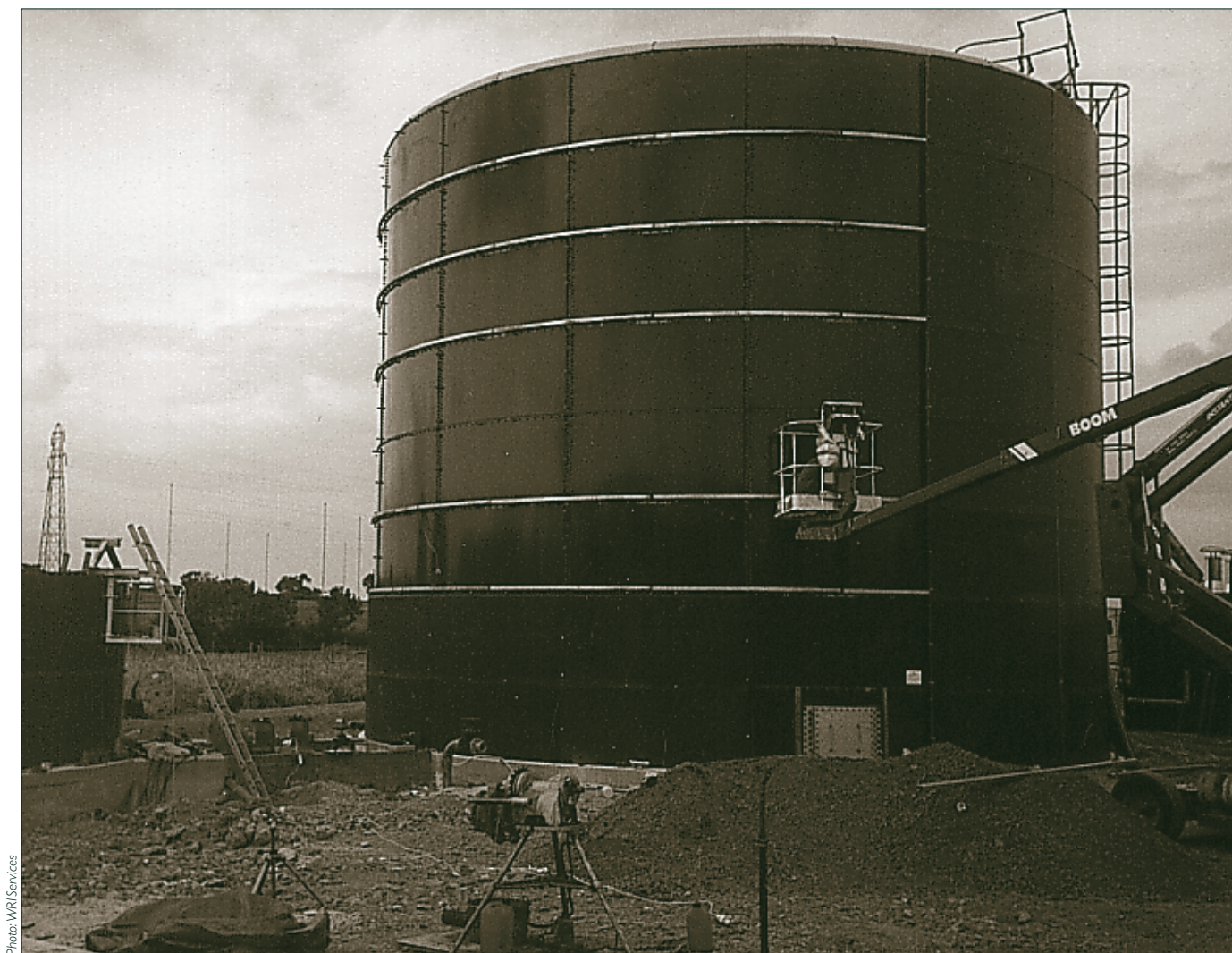
Digester under construction.
